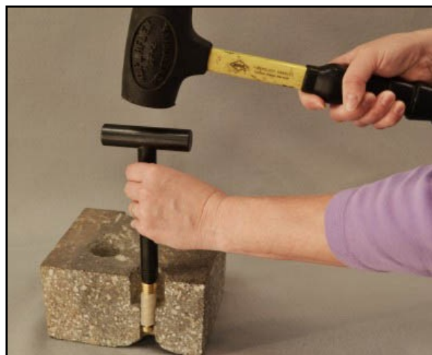
Figure 2. Flush-Mount Installation Process.
