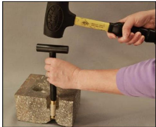
Figure 2. Flush-Mount Installation Process.
