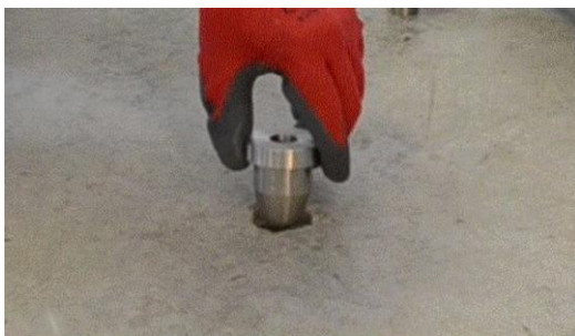
Figure 3. Testing Depth with the Drilling Guide
