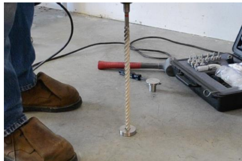
Figure 4. Using the Drilling Guide
